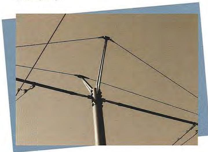
The "grooved" design and surface work on the lower part of the posts takes accidents into account and limits the traces left by vehicle impacts. The use of cast iron lends subtlety and harmony, whilst noticeably reducing the diameters at the top and bottom of the post, compared with steel.
