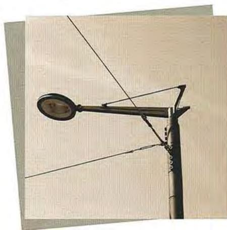
Whether transverse, central, lateral, strainers, according to their fitting, with sleeves or single or double stayed arms, all these supports have different functions: signage support, banners, street lighting...
